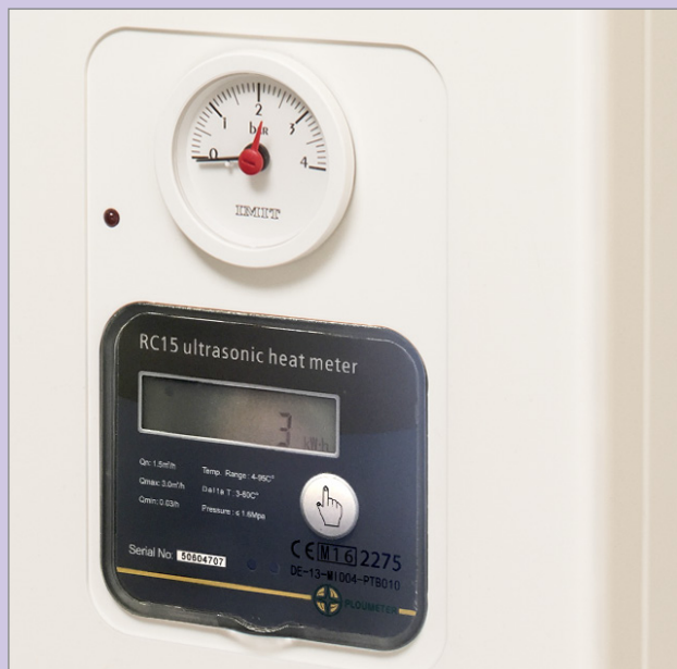
Our ModuSat® heat interface units feature an integrated MID certified energy meter as shown above.
